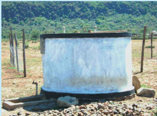
Water treatment and regulation tank in Kailer
